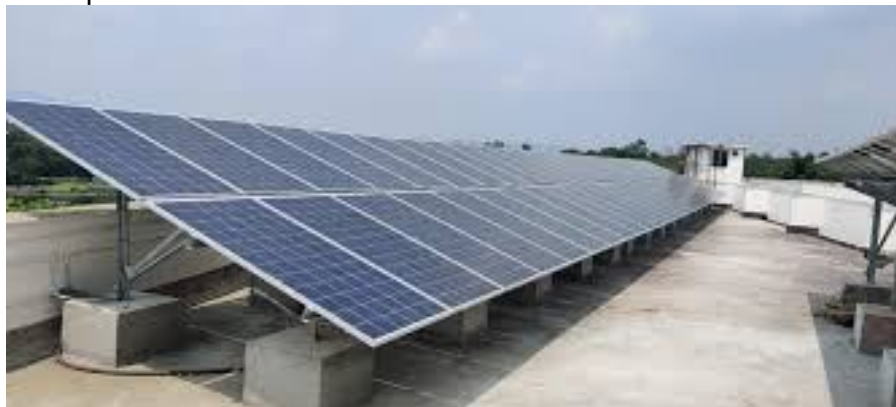
Figure 7 : A Solar roof top system
